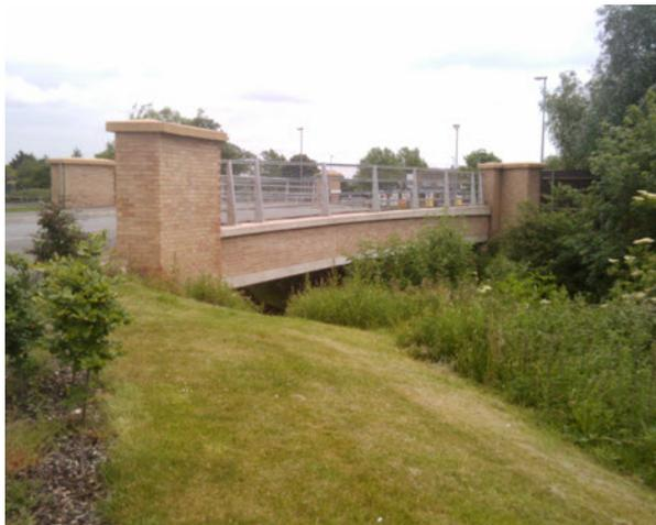
The design consisted of adapting an existing large four armed roundabout to incorporate a fifth arm to serve the new residential development. This new access arrangement required a new adoptable access road, and a 20 m long road bridge constructed over the River Cole.
